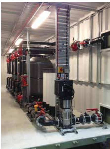
Waterco’s Micron fiberglass filters are made from continuous strands of high quality fiberglass filament wound under controlled tension to create a seamless, impervious vessel.
