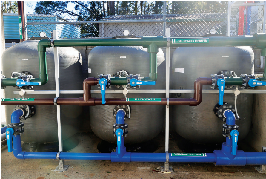
To ensure consistently clean and hygienic water for students and teachers, Gerrie Baldwin from Baldwin Aquatic decided to install Waterco's Micron Commercial Fibreglass Filters (3 x SMD1200).
