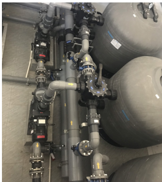
Waterco’s SM1200 Micron Media Filter (side mount) and Hydrostar MKIV Pumps.
