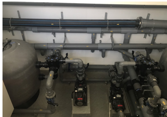
Waterco’s SM1200 Micron Media Filter (side mount) and Hydrostar MKIV Pumps.
